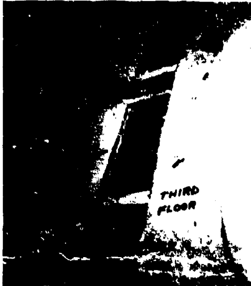
Figure 4.67 Post-Dogwood, -Olive, and -Pine, (Item 26) Station 3.1.1, crack in third floor at intersection of front wall between Column Line 11 and south shear wall. Pres- sure levels: Dogwood, 12 psi; Olive, 8.4 psi; and Pine, 13 psi.
